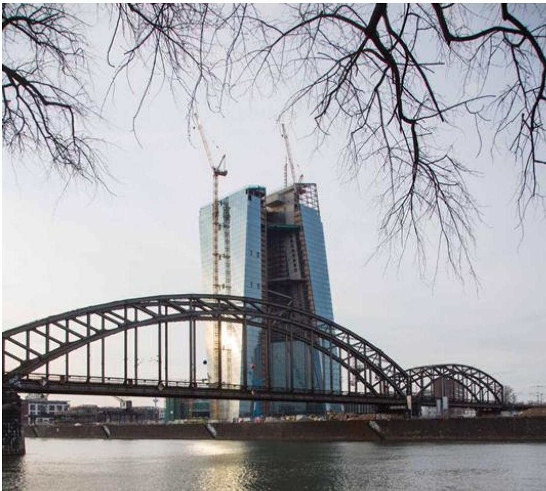
The new European Central Bank headquarter in Frankfurt/Main under construction
